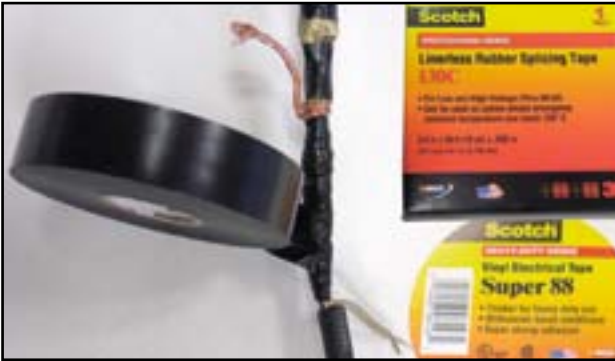
Stretch it out and cover with three layers of Scotch 130C tape, and three layers of Scotch Super 88 PVC tape.
