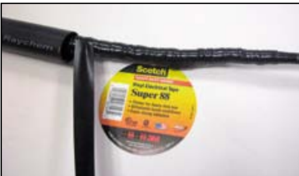
Repeat with three coverings of Super 88 PVC tape.
