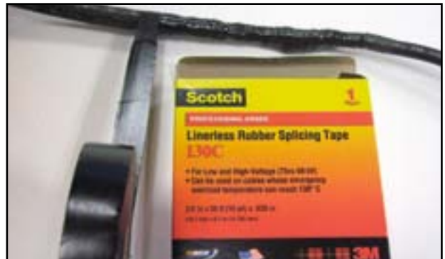
Stretch it out and tape both together with three coverings of Scotch 130C tape, extending onto the cable itself each side.
