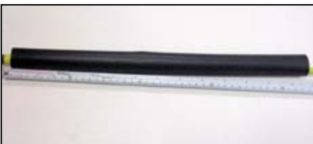
Slide a tube over the join.
