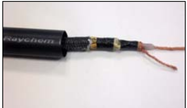
6 Slide an approximately 40cm shrink tube onto the cable.
